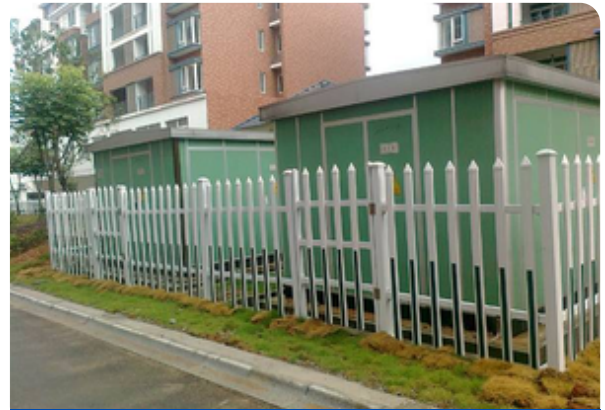
Power Station Fencing
